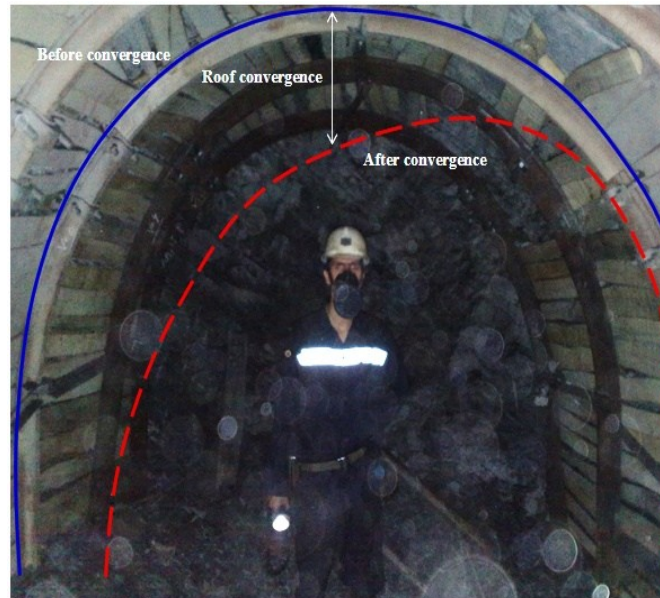
Figure 8. Comparison of the main gate roadway situations before and after convergence, Parvade-2 coal mine [9].
