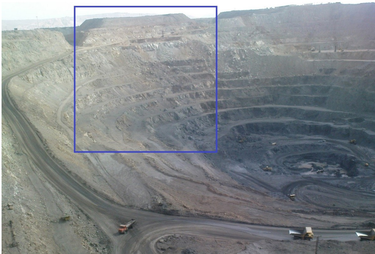
Figure 14. The failure in the old pit Tectonic Block I [54].
