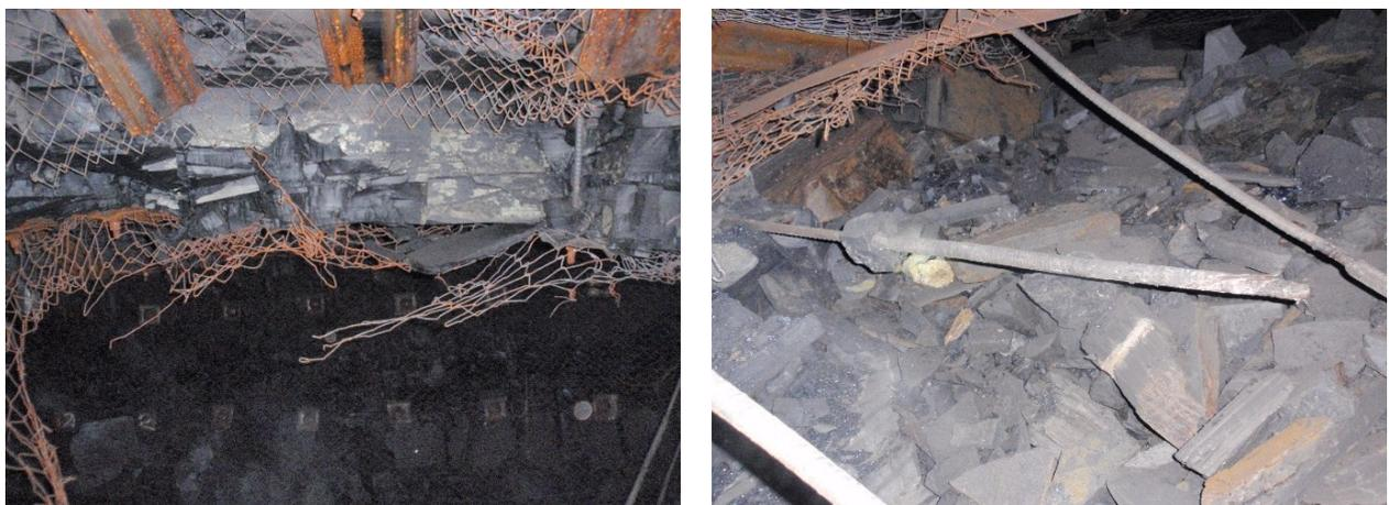
Figure 3. Failure mode of longwall installation roadway.
