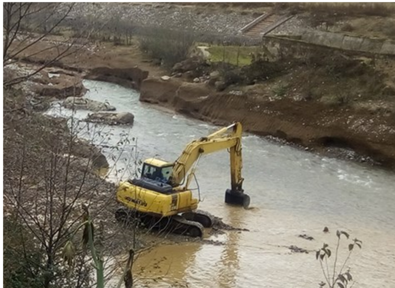
Figure 1. Excessive extraction of river bed materials.
