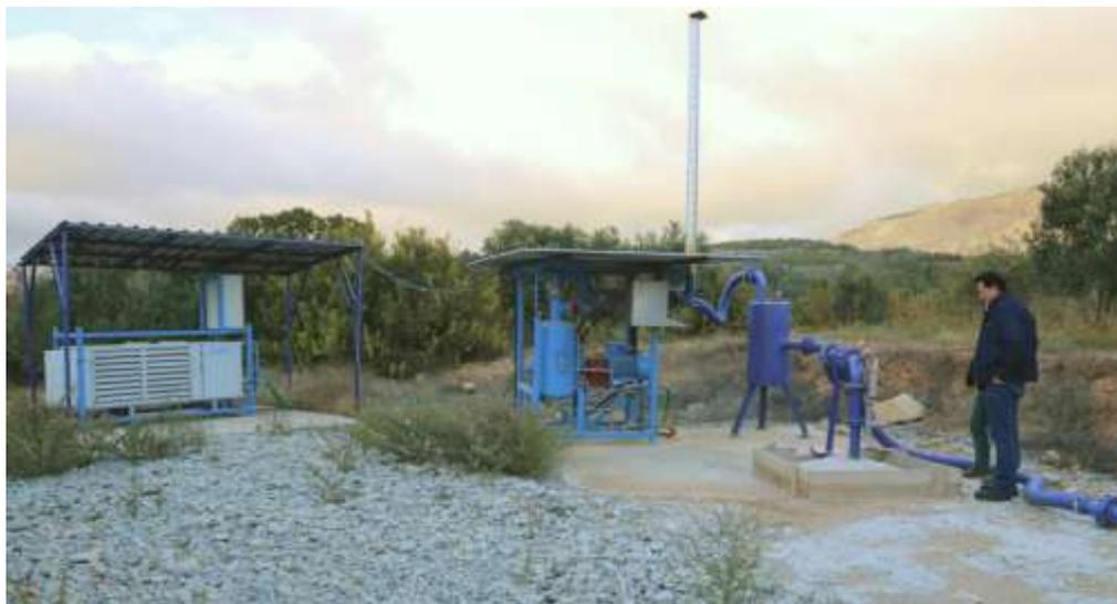
Figure 7. Methane drainage borehole and facility above Panel A.
