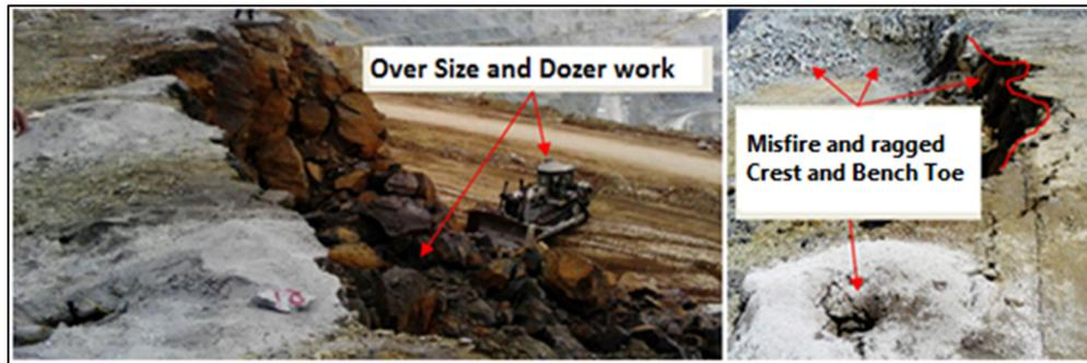
**Figure 6. A sample of a previous blast and the destructive events after the blast.**
