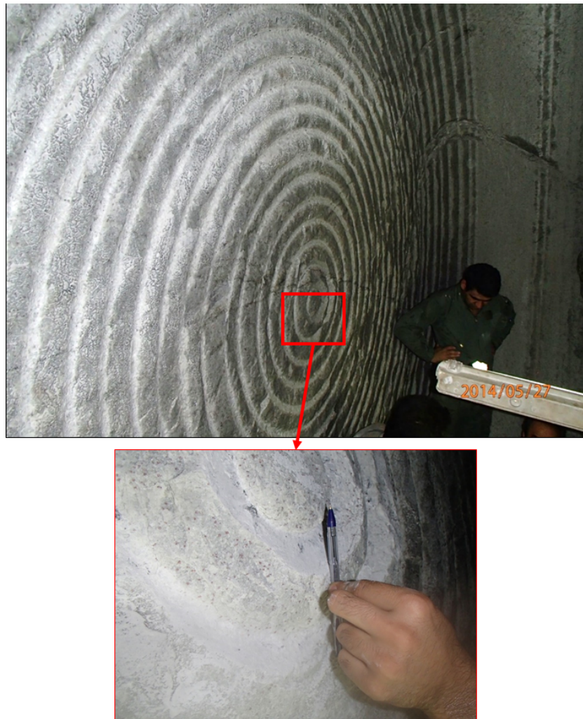
Figure 8. An example of a tunnel face in a part of the tunnel, where grinding was dominant. The creation of ridges and adjacent deep grooves are indications of an incomplete chipping [35].
