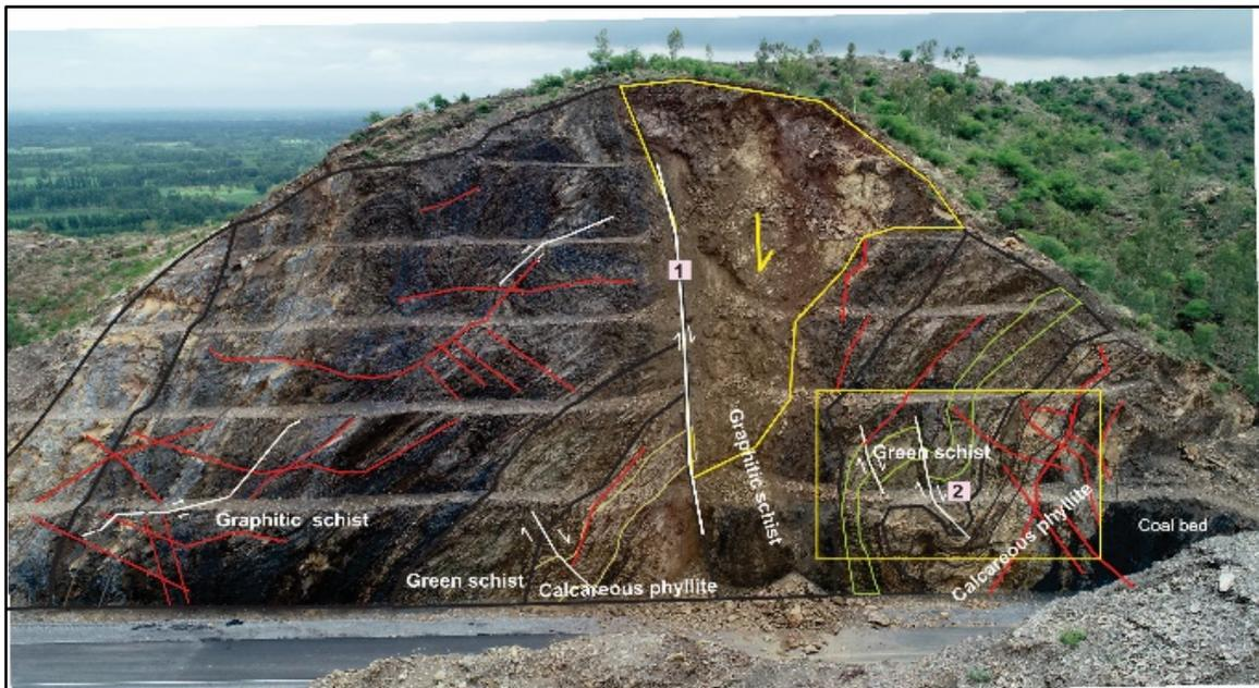
**Figure 3. Unstable rock cut slope prone to failure at KM-37 of the Swat motorway.**
