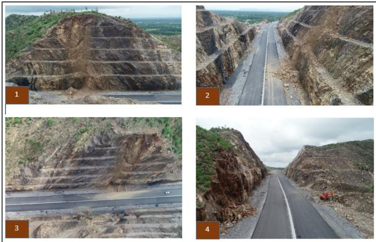
Figure 1. Unstable rock cut slope at KM-37 section of the Swat motorway.
