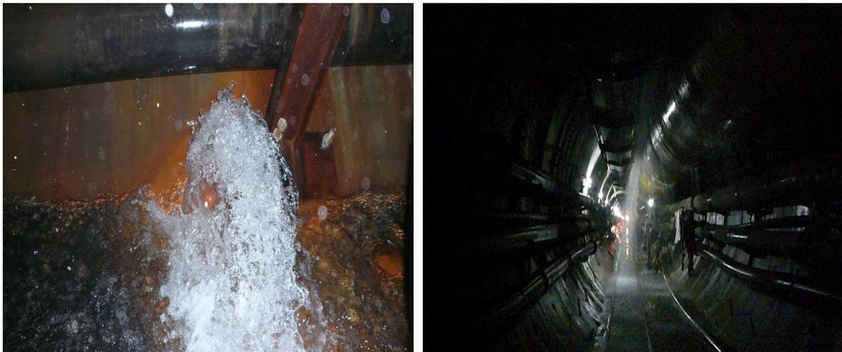
**Figure 18. Inrush water in Nosoud tunnel.**
