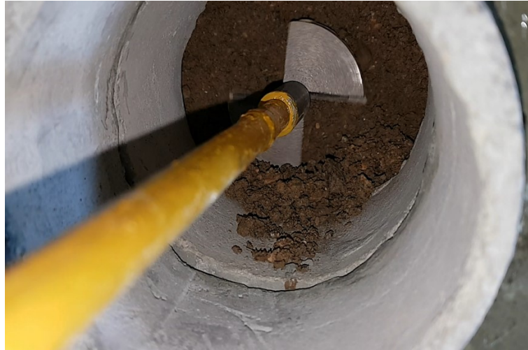
Figure 12. Mechanized drilling and simultaneous segmentation.
