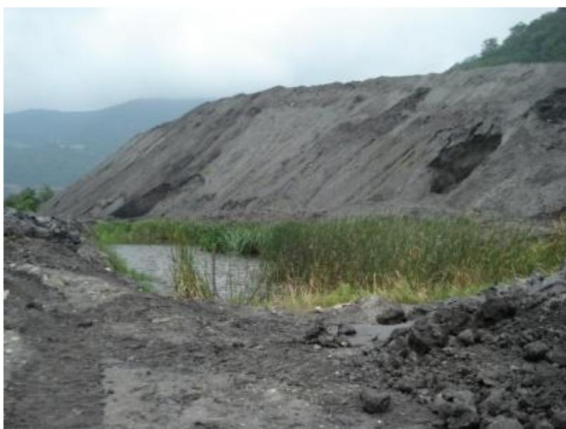
Figure 2. Accumulation of a large amount of waste in Zirab coal washing plant.
