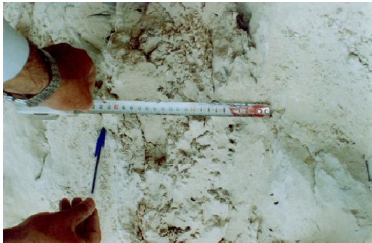
Figure 1. Fault thickness in Kangir Dam, Iran.
