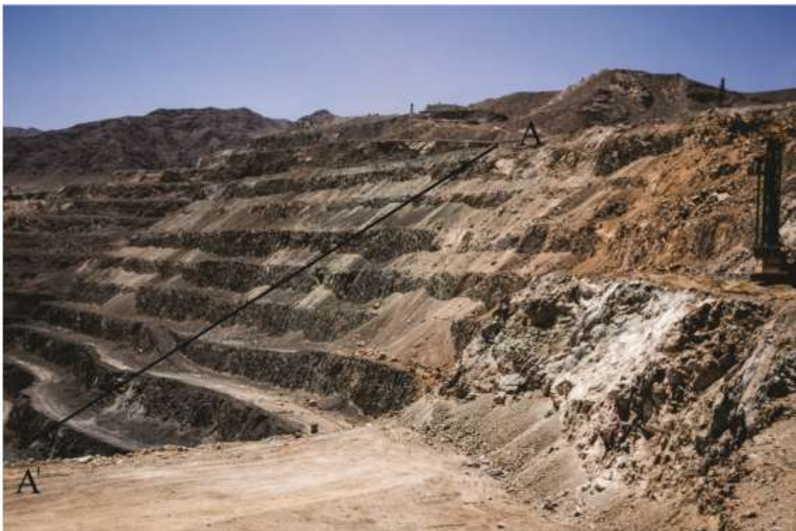
Figure 3. The approximated trace of the section under study (AA') on the NW slope of Chadormalu mine.
