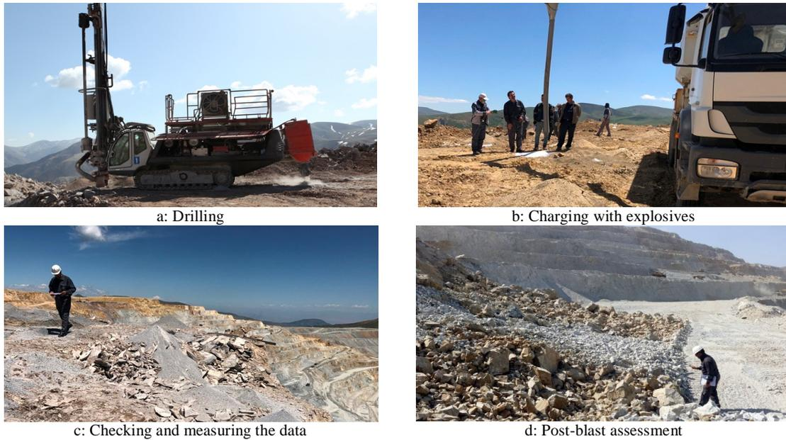
**Figure 3. Blasting cycle and measuring the field data**
