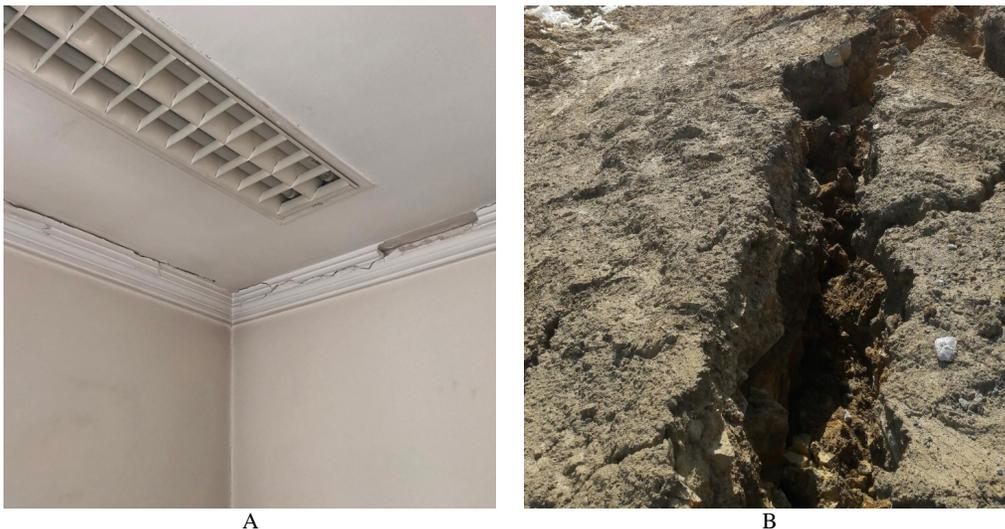
**Figure 4. Damages caused by blasting in the (a) structures and (b) environment around of the Sungun copper mine.**
