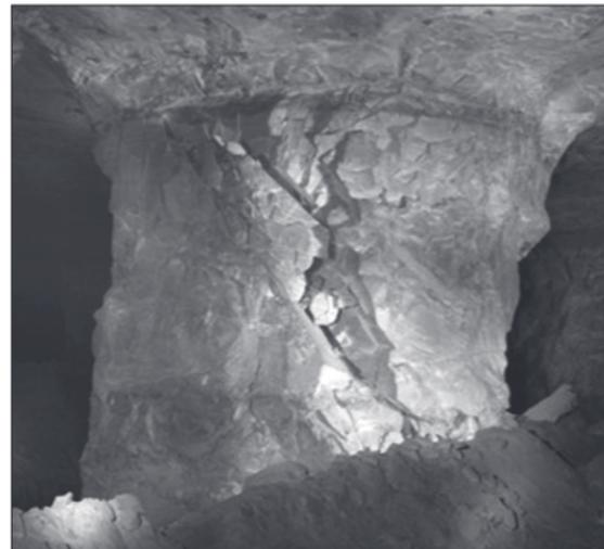
**Figure 1. Sliding along two non-persistent joints in a pillar (Esterhuizen, [2]).**
