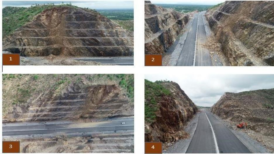
Figure 2. Failure of slope at 37 Km chainage of Swat motorway.
