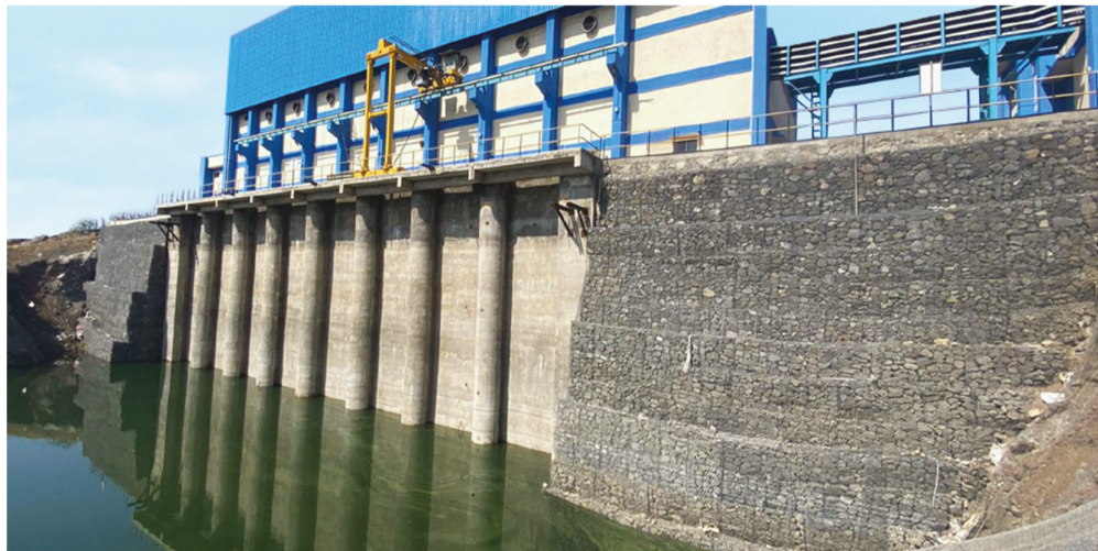
Figure 8. Gabion wall after completion submerged under backwater.
