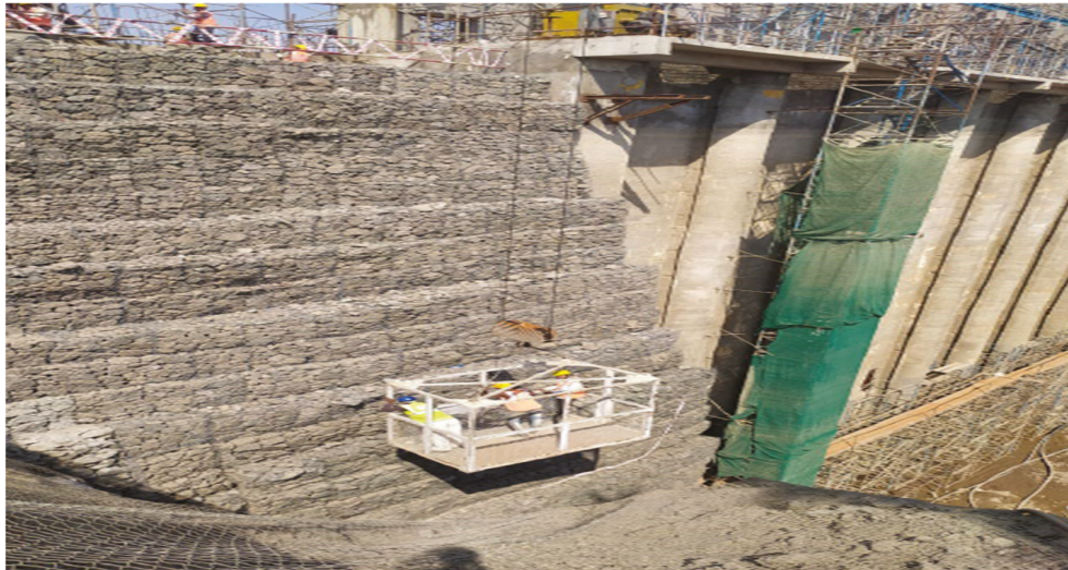
Figure 7. Mobilization of boulders using basket attached to the crane.
