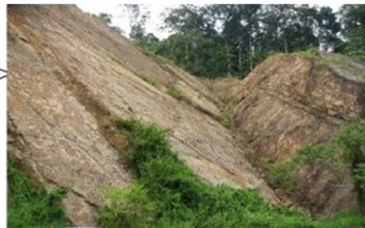
Figure 6. Wedge Failure [30]
