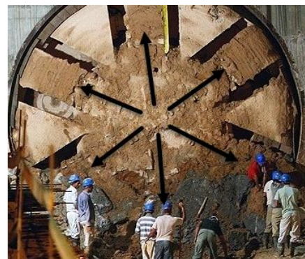
(c) Line 1 of Ahvaz Metro Project
