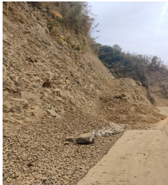
Figure 1. Image of the studied slope.
