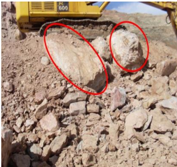
Figure 3. Boulders produced as a consequence of blasting activities at the Anguran mine [16]
