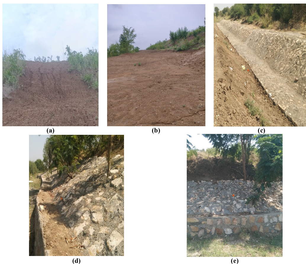
Figure 10. Implemented remedial measures at the site
